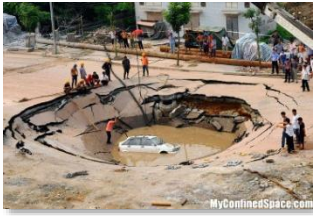
Sinkholes are big.
